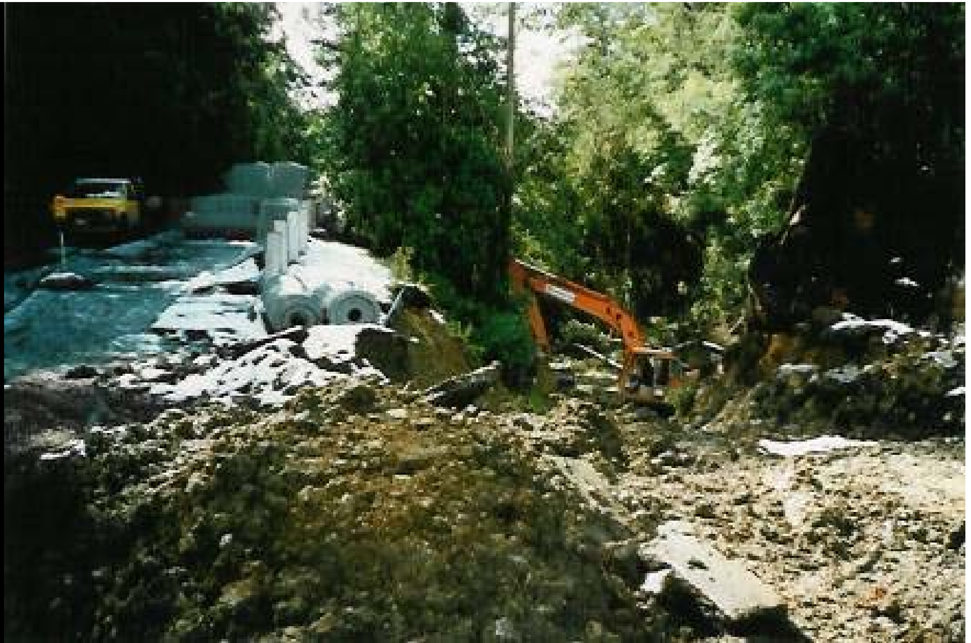
The engineering clean up (Strickland Avenue 1996)
