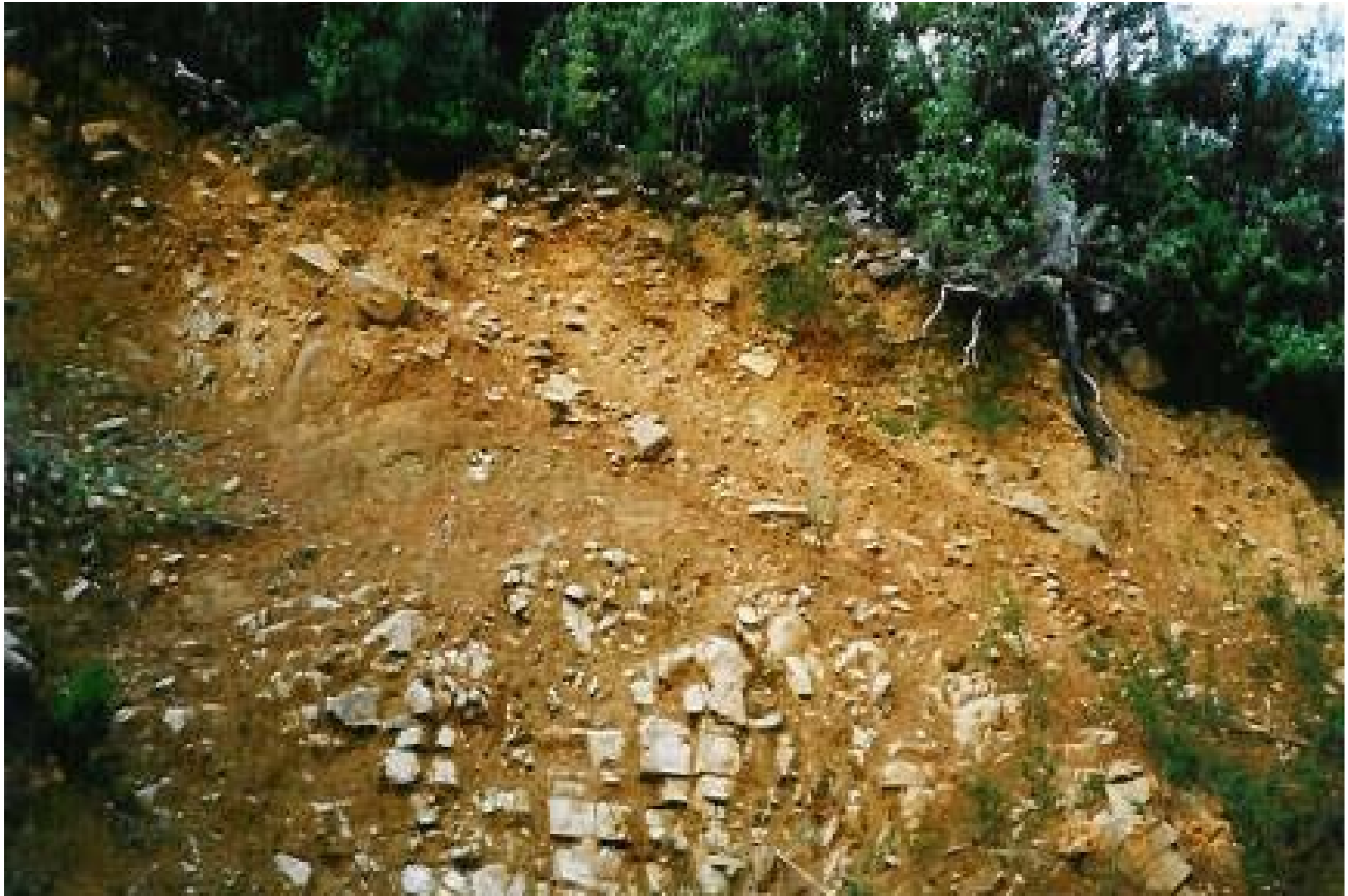
Future scope for failure – nature of materials (west Mt Wellington)
